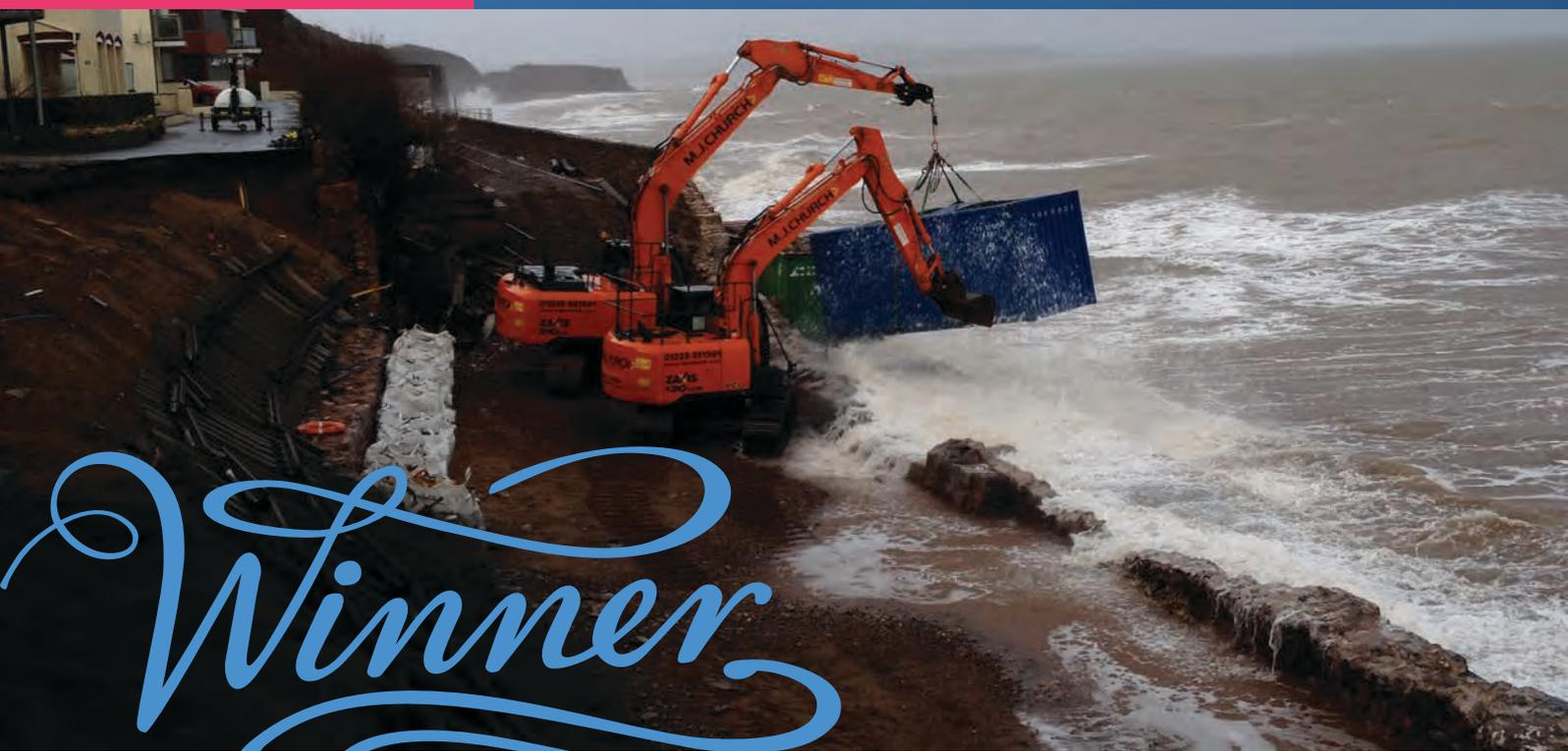
Emergency repairs at Dawlish presented many challenges for Network Rail, including the need to stabilise a massive sea cliff after failure caused by the intense rainfall in the storm conditions. The project team's innovative solution – deliberately initiating a landslide – was crucial in getting the line open again, as well as earning the team the APM's Project of the Year award.
